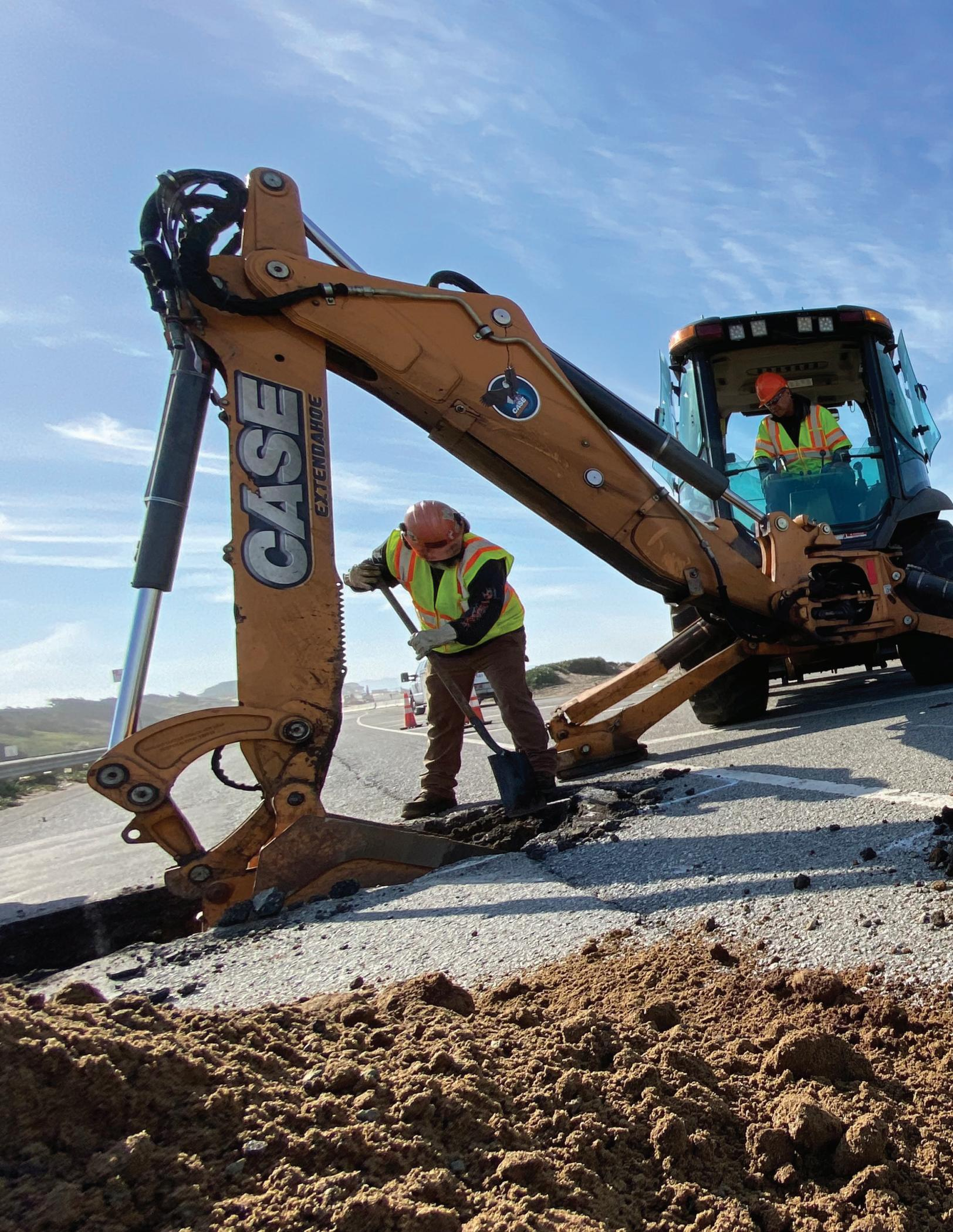
Crews from the Bureau of Street and Sewer Repair dig two holes to provide access for our engineers to see beneath the pavement.
