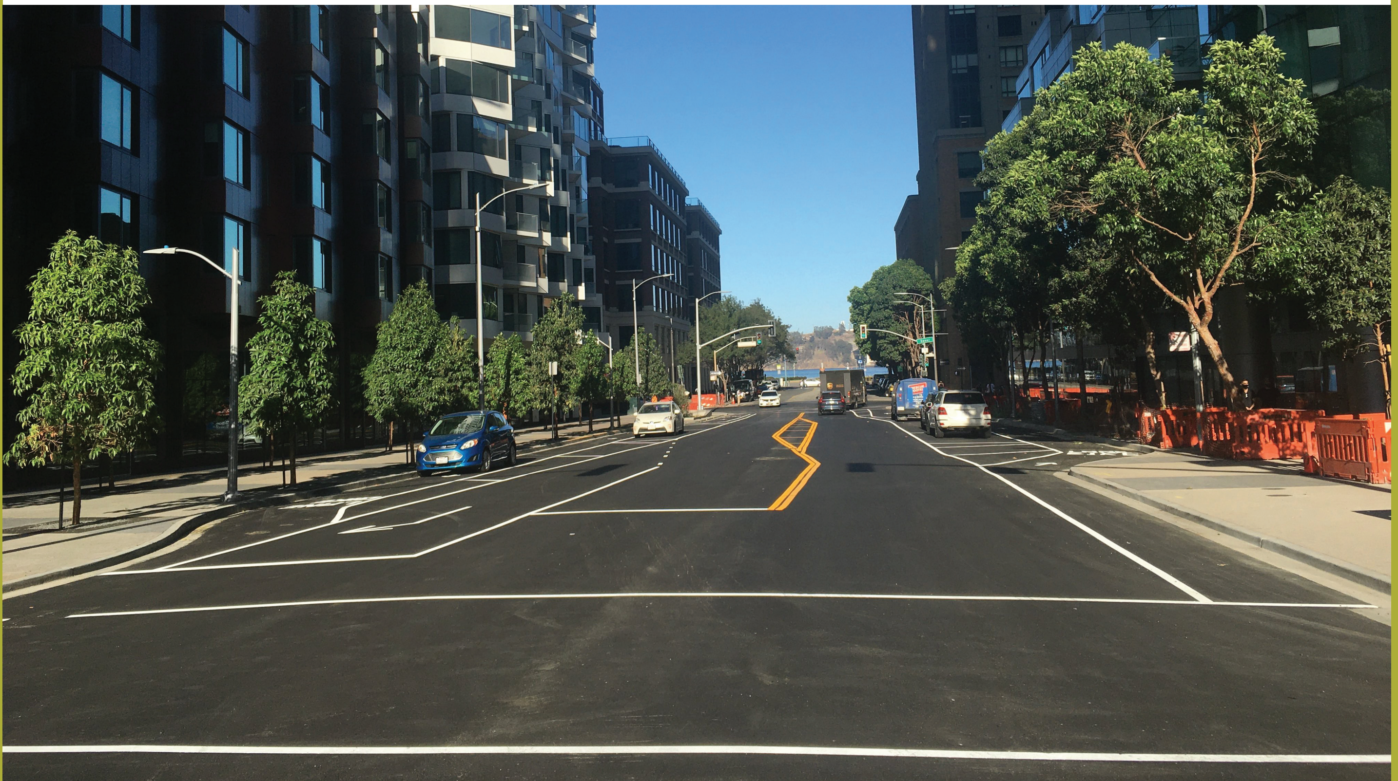
After the hot asphalt goes down, traffic striping is applied.
