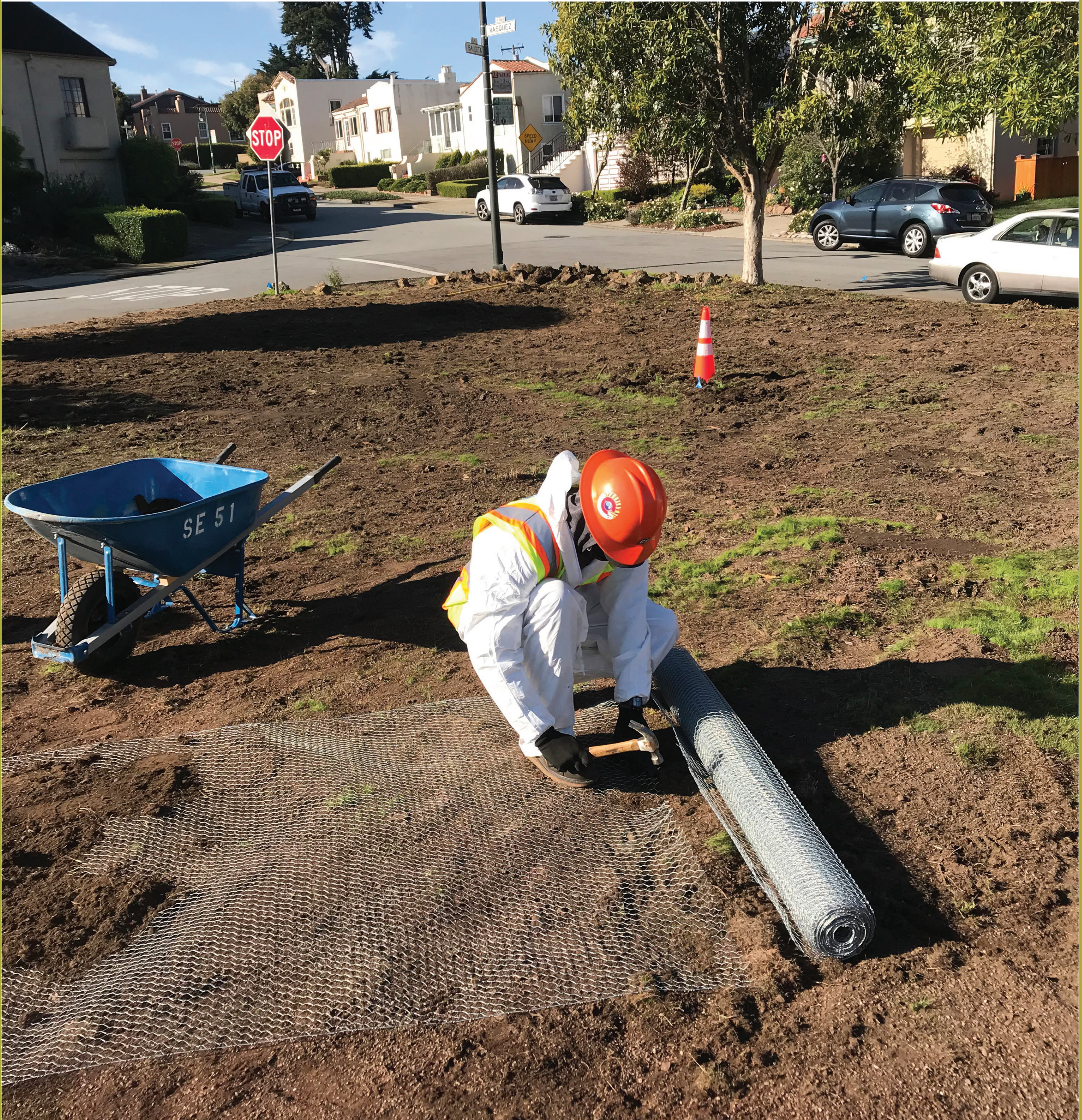
A Bureau of Urban Forestry landscaper lays down gopher wire at Triangle Park.
