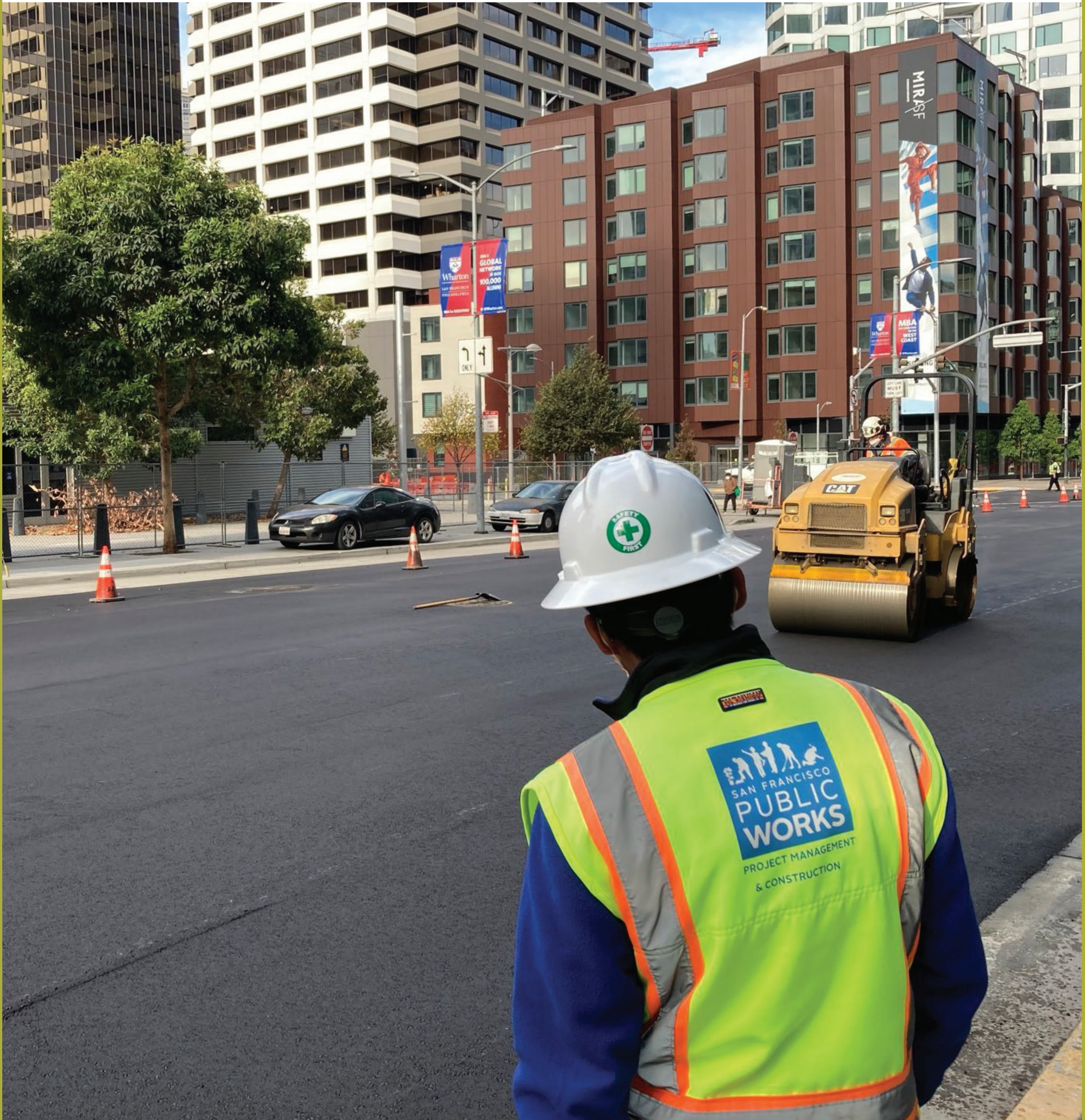
A road roller smooths out the freshly paved Folsom Street roadway.
