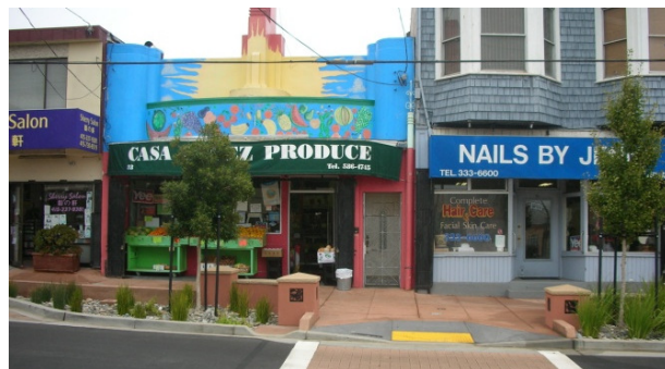
Bioretention planter and landscape
