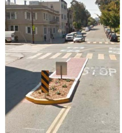
Raised island with mountable section for driveway and emergency vehicle access
