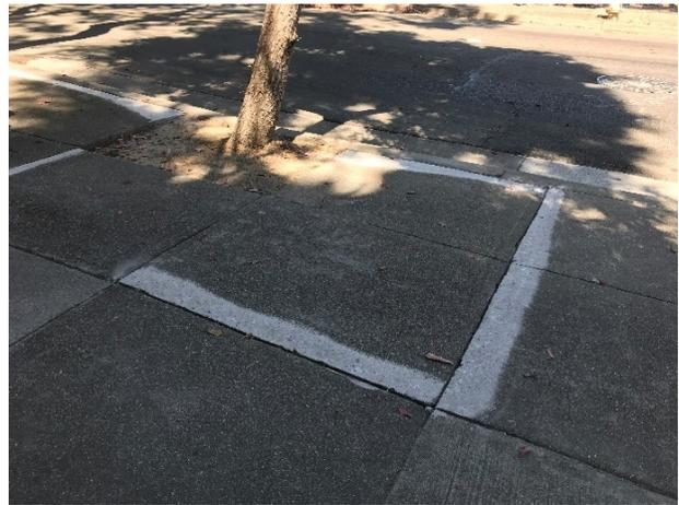
Sidewalk after being treated by concrete slicing.
