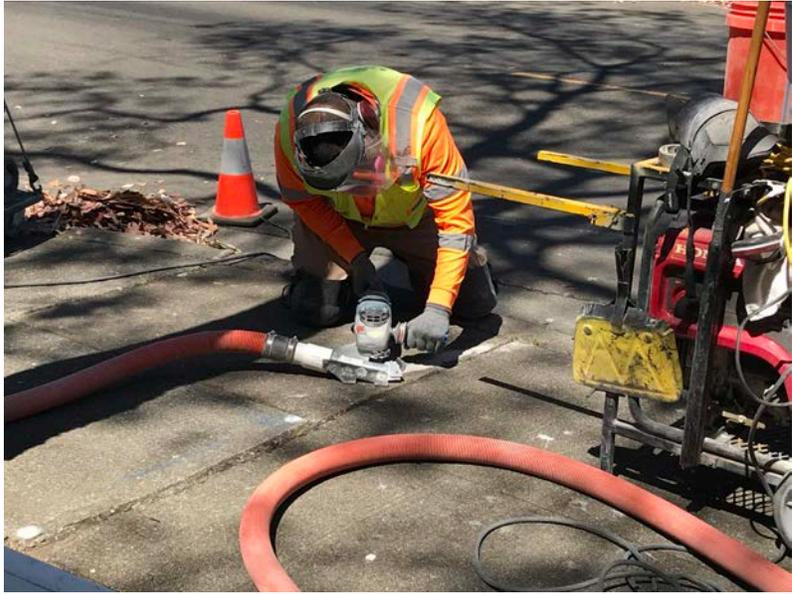
Concrete slicing is a fast, cost effective and environmentally friendly repair method that does not require removal and replacement of sidewalk squares.
