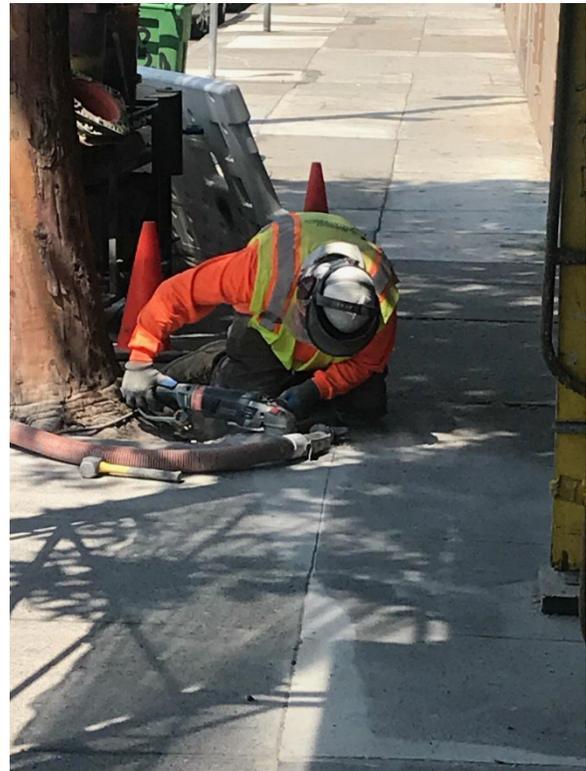
The use of concrete slicing has sped up sidewalk repairs and improved pedestrian safety in many neighborhoods.
