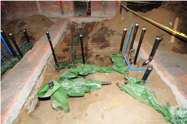
Under-slab utilities installation at Fire Station 30
