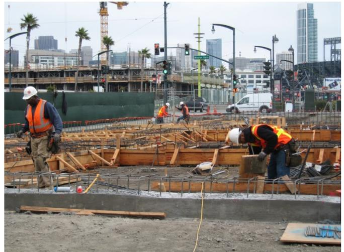
Grade beam construction at Level 1
