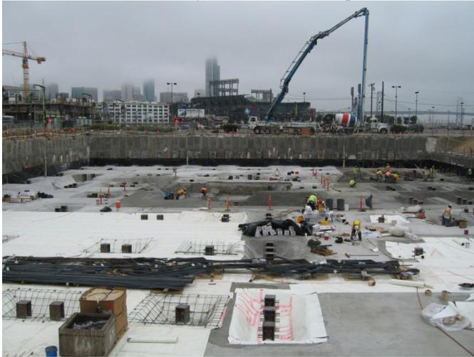
Construction activities at Basement level: mud-slab pour; protection slab installation; subgrade waterproofing; reinforcement at pile caps
