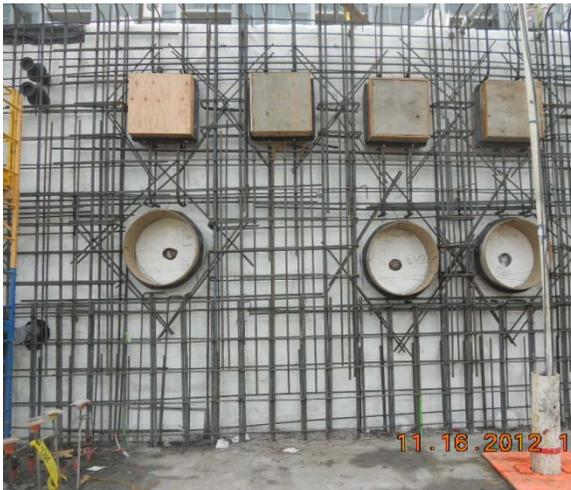
Block-outs for penetrations at basement wall
